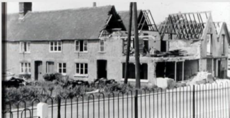
1966 Demolition of old bakery
